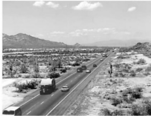
Level of Service "B"
